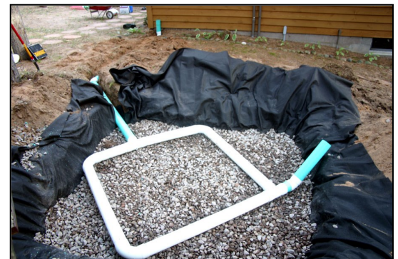
Infiltration Pit Under Construction
