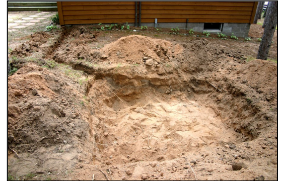
Infiltration Pit Dug to Capture Roof Runoff Water
