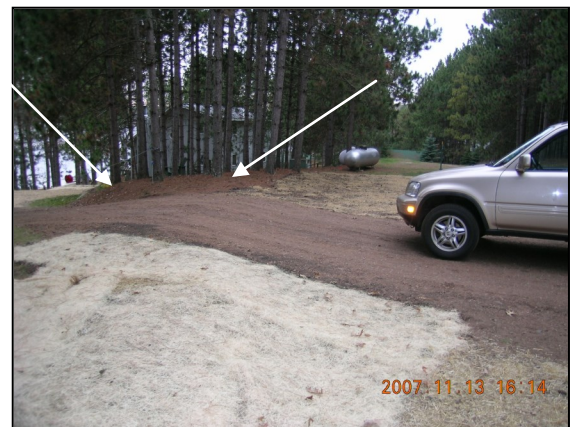
Berm Keeps Water from Eroding the Slope to the Lake
